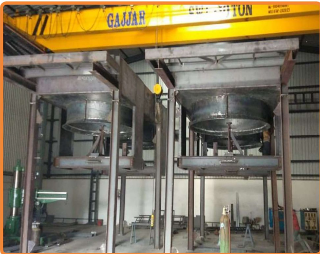
BASE STRUCTURE OF AIR COOLED HEAT EXCHANGER
